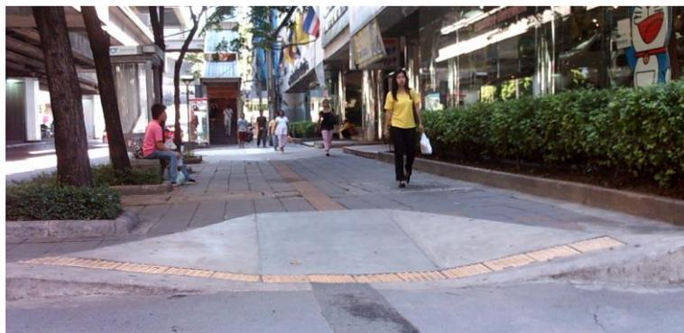
Photo 2-2. Clear and leveled approach with Kerb Ramps
