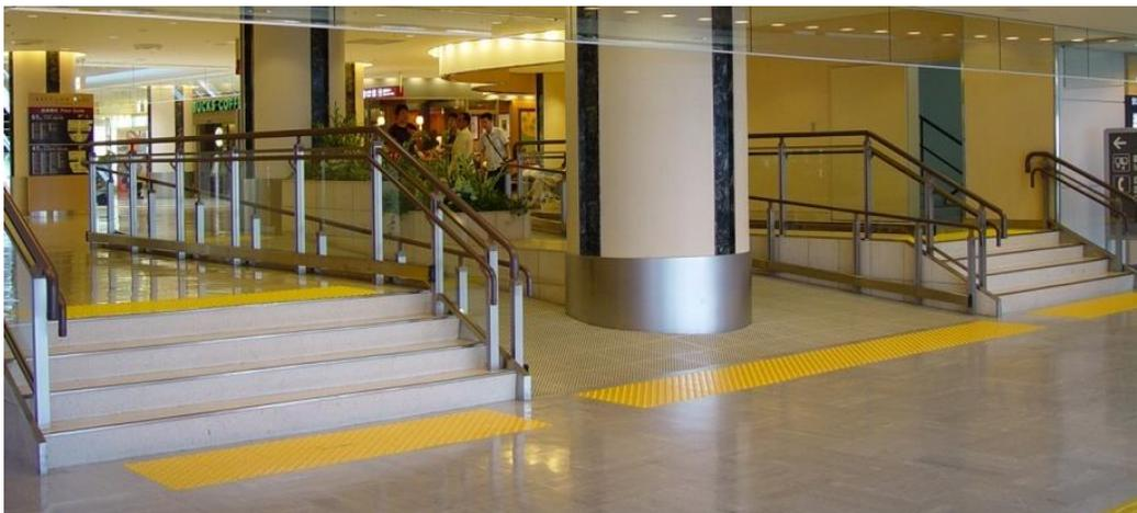
Photo 8-1. Accessible elements with colour contrast interiors
